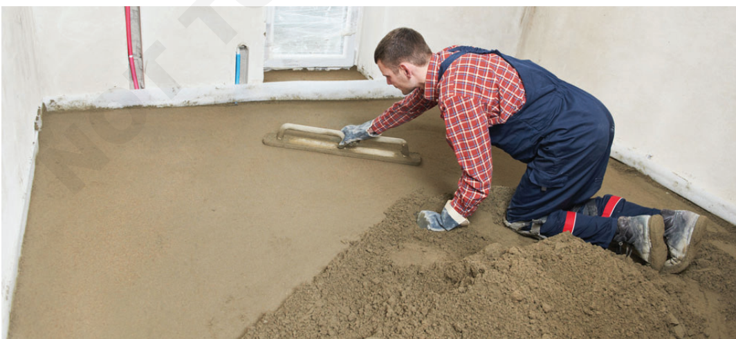
Casting screeds in ground of site
