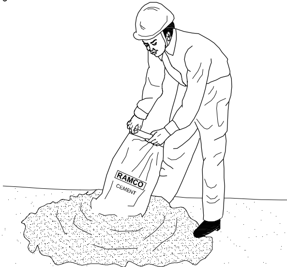
EMPTYING CEMENT BAG
