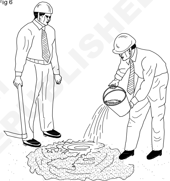
ADDING WATER IN DRY MIX
