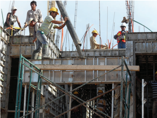
Placing the concrete (By Mechanicla) and Compaction
